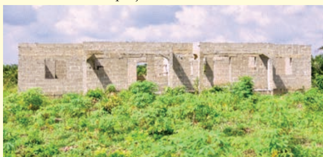
Rector's Lodge under construction by Yaba Baptist Church, Lagos.
