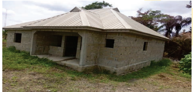
3-Bedroom flat under construction by the three Lagos Baptist Conferences
